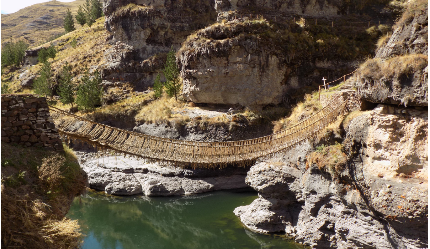
ABOVE: The author went to Peru to see the Q'eswachaka Bridge, which has been rebuilt annually for the past 500 years. Its makers use the composite technique (Photograph by the author).
