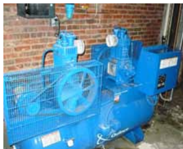
NEW AIR COMPRESSOR
