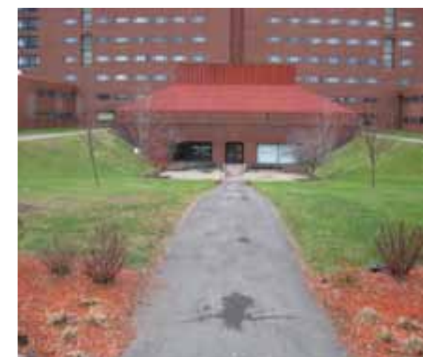
THE EXTERIOR RAMP TO FACILITY IS NOT ADA COMPLIANT.
