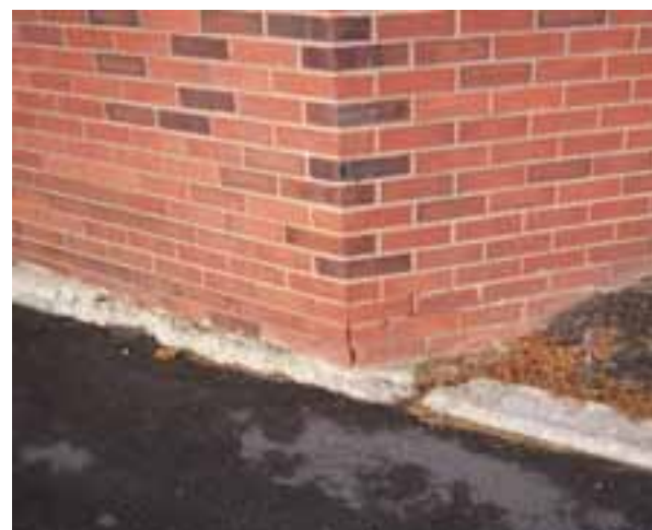
CRACKS IN EXTERIOR BRICK WALL
