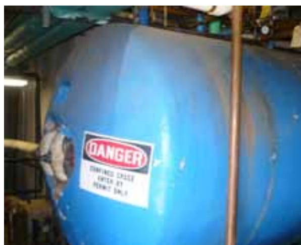
HOT WATER STORAGE TANK
