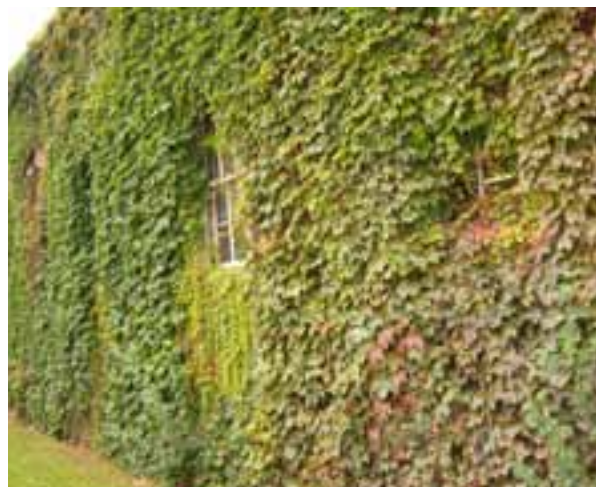
DENSE GROWTH OF IVY ON EXTERIOR WALLS.
