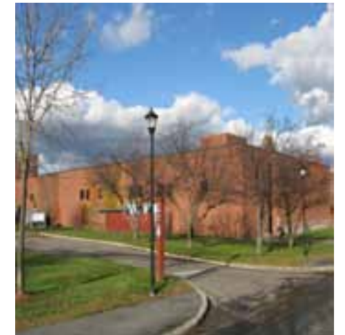
NO CURB CUTS AT SIDEWALK/ROAD INTERSECTION
