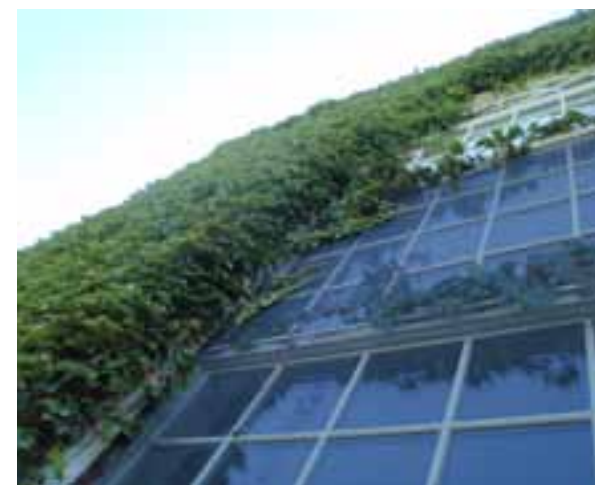
IVY GROWTH ON EXTERIOR WALL
