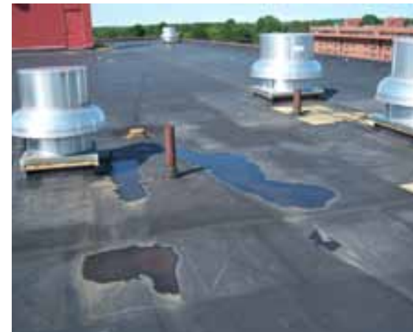
HIGH ROOF HAS MANY PATCHES AND THERE IS SOME PONDING IN AREAS
