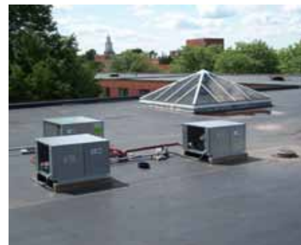
VIEW OF ROOFTOP EQUIPMENT.
