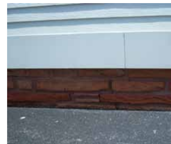
EXTERIOR CUT STONE FOUNDATION.
