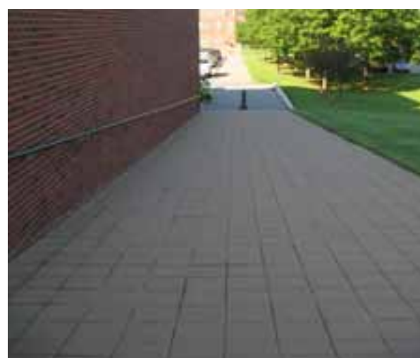
EXTERIOR ACCESS TO THE PLAZA IS VIA RAMPS. THE RAMPS ARE SLOPED GREATER THAN 1:12.
