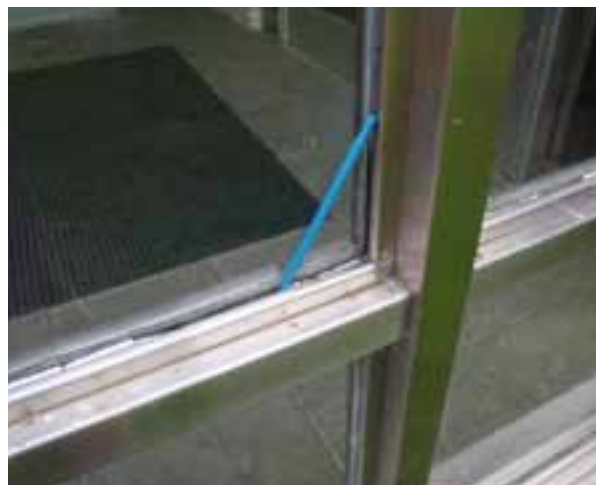
DETERIORATING SEALANT AT THE WINDOWS
