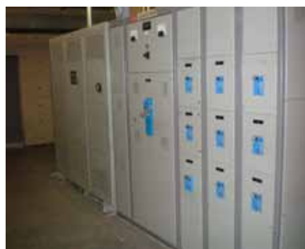
CRANE COMPLEX: NEW ELECTRICAL SWITCHGEAR
