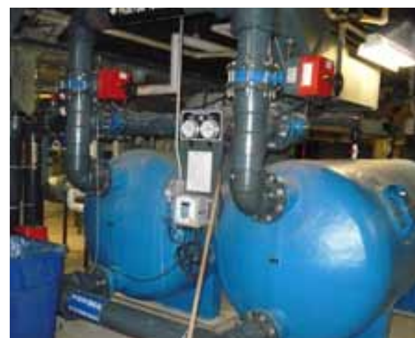
NEW POOL FILTRATION SYSTEM
