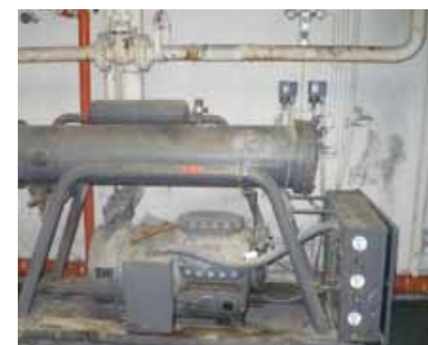
OLD CHILLER AND MECHANICAL ROOM
