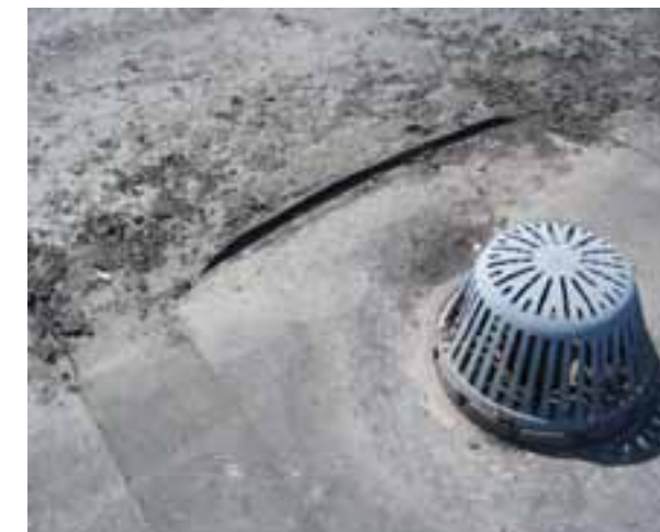
VIEW OF ROOF THAT ARE IN DETERIORATED CONDITION WITH DELAMINATED SEAMS
