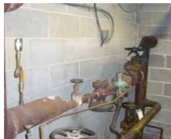
UN-INSULATED HIGH PRESSURE STEAM ENTRANCE AND PRESSURE REDUCING STATION
