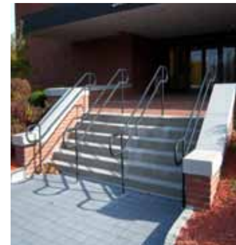
EXTERIOR STAIR AT SNELL THEATER
