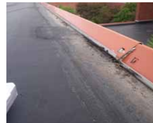
BUILDING PERIMETER - POSSIBLE WATER INFILTRATION INTO THE EXTERIOR WALL CAVITY.
