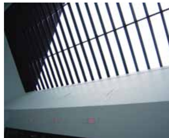
INADEQUATE MOISTURE CONTROL AT THE SKYLIGHT IN THE LOBBY.
