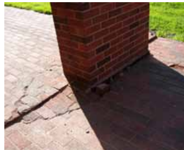
THE PAVING ADJACENT TO THE BUILDING IS IN POOR CONDITION.
