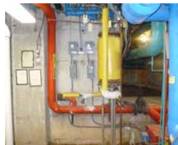
PIPING IN MECHANICAL ROOM
