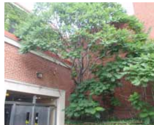
THERE ARE SHRUBS AND TREES GROWING TOO CLOSE TO THE BUILDING
