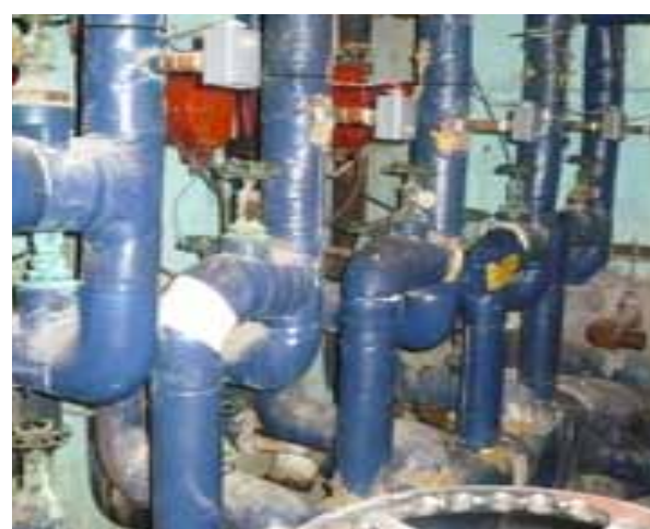
RADIATION ZONE PUMPS
