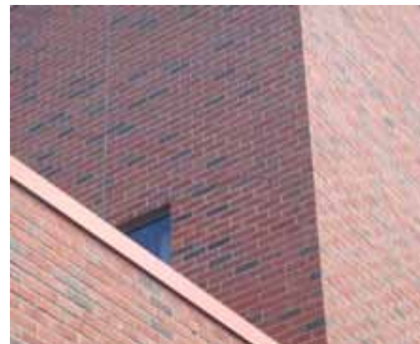
THE BRICK MASONRY IS IN GOOD CONDITION.
