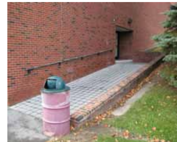
EXTERIOR RAMP'S SLOPE IS GREATER THAN 1:12 AND ONLY ONE HANDRAIL.
