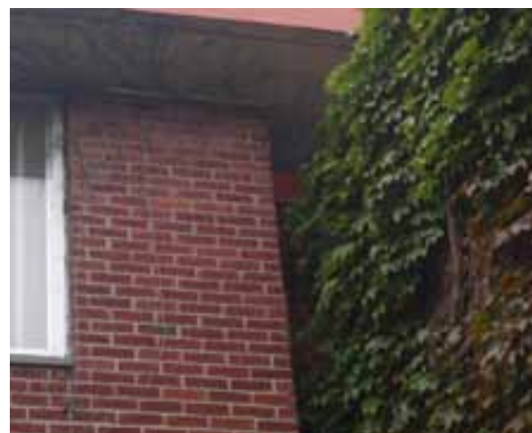
IVY GROWTH ON EXTERIOR WALLS.
