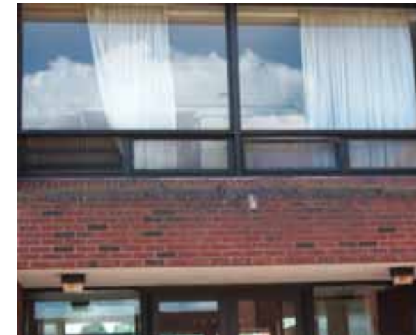
EXTERIOR ENVELOPE MASONRY STAINING.
