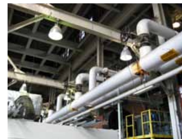
VIEW OF STEAM HEATERS
