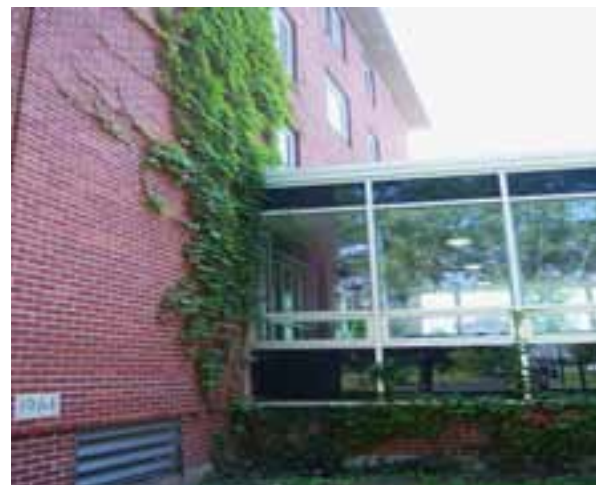
IVY GROWTH ON EXTERIOR MASONRY WALL.
