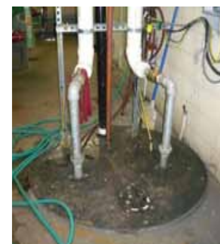
SEWAGE EJECTOR PUMP
