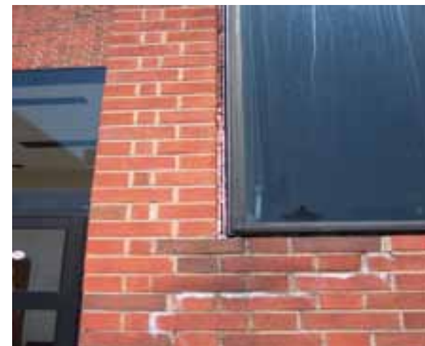
CRACKS IN THE MASONRY ALONG THE BAND OF WINDOWS ON THE WEST
