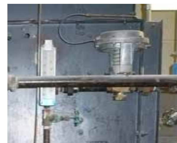
PIPING AT AIR HANDLING UNIT
