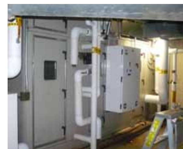
NEW AIR HANDLING UNIT
