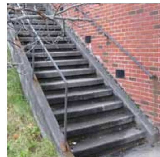
THE EXTERIOR RAMP IS MISSING HANDRAIL EXTENSIONS.
