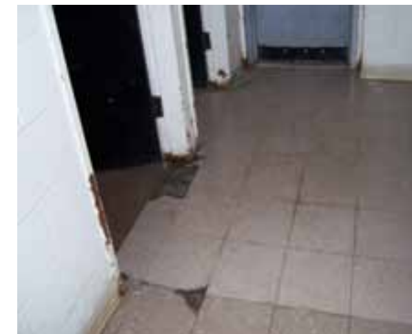
SOME OF THE FLOOR FINISHES APPEAR DATED.
