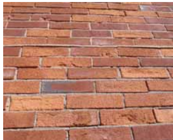
SPALLING AND MORTAR JOINT ISSUES.
