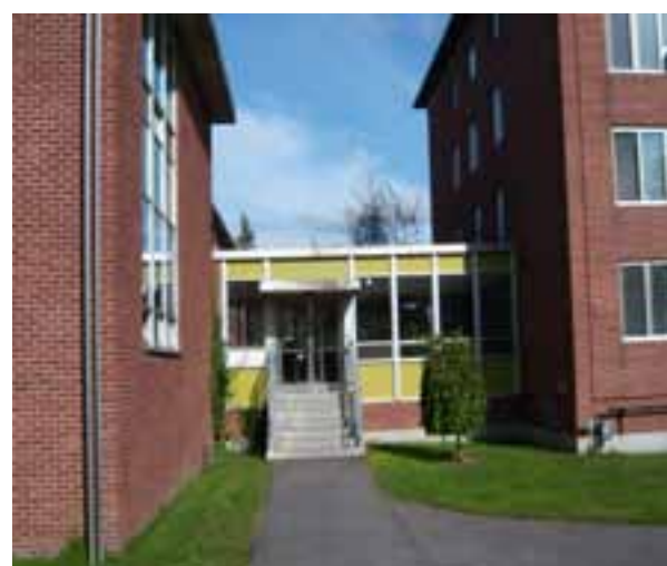
ENTRANCE IS NOT WHEELCHAIR ACCESSIBLE
