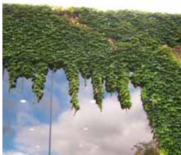
IVY GROWTH ON EXTERIOR WALL AND GLAZING
