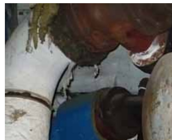
POOR INSULATION ON STORM PIPING
