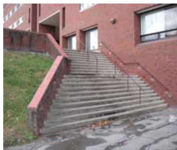
EXTERIOR STAIRS TO PLAZA AT RESIDENTIAL HALL ENTRY DOES NOT HAVE
