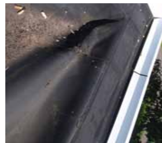
EPDM MEMBRANE BUCKLING.
