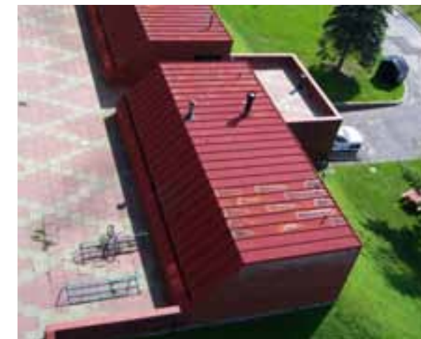
THE UPPER ROOF IS METAL WITH STANDING SEAMS.
