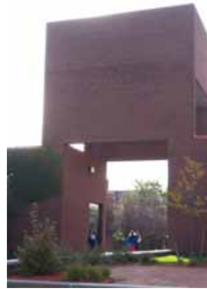
EAST QUAD TOWER
