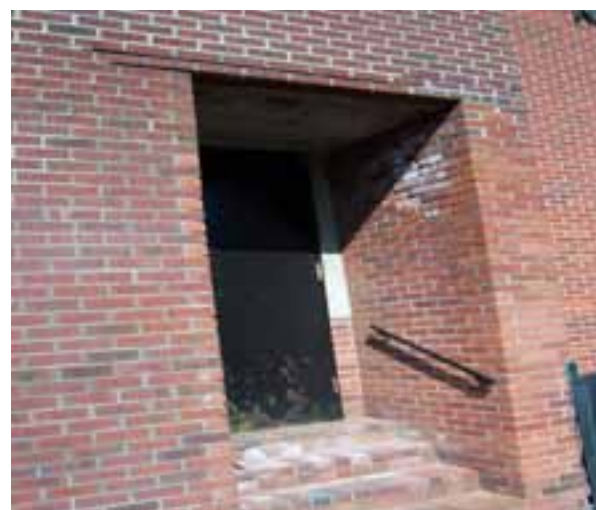
EXTERIOR MASONRY STAINING AND EFFLORESCENCE. EGRESS EXIT NOT TO CODE.
