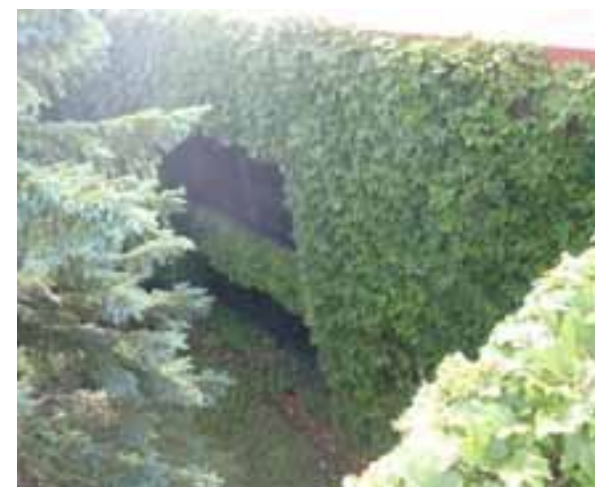
IVY GROWTH ON EXTERIOR NORTH MASONRY WALL.
