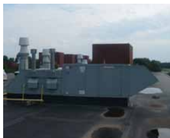
MAKE-UP AIR UNIT AND FUME HOOD EXHAUST FANS
