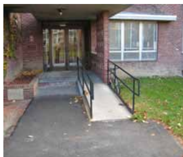
SISSON'S MAIN ENTRANCE IS WHEELCHAIR ACCESSIBLE WITH A RAMP BUT THE RAMP'S WIDTH IS NON-COMPLIANT.
