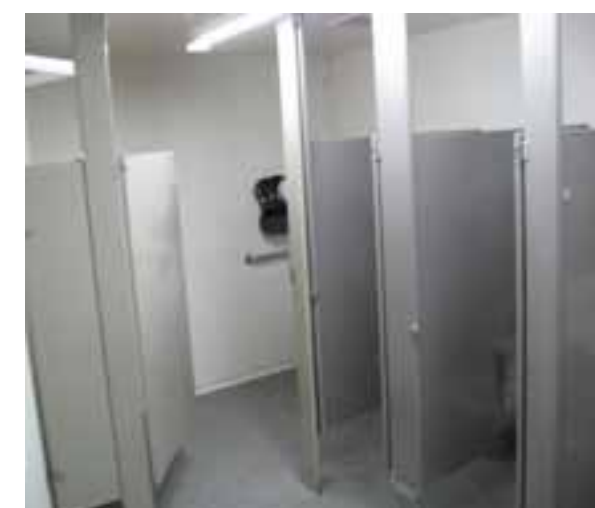
PUBLIC TOILET ROOMS AT LOWER FLOOR ARE ADA-COMPLIANT.
