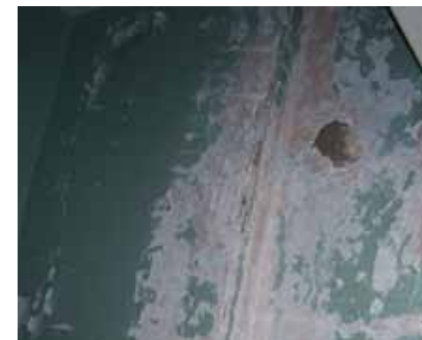
INTERIOR DAMAGE TO WALLS.
