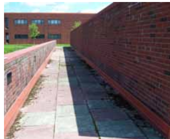
LOWER ROOF FORMS A PLAZA FOR BOWMAN HALL; IT IS FINISHED WITH PAVERS.
