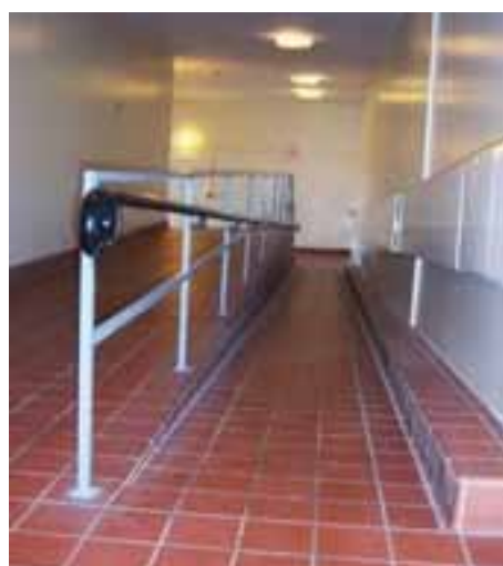
THE RAMP INSIDE THE MAIN ENTRY CONTAINS ONLY (1) HANDRAIL, AND IS LESS THAN 40" WIDE.
