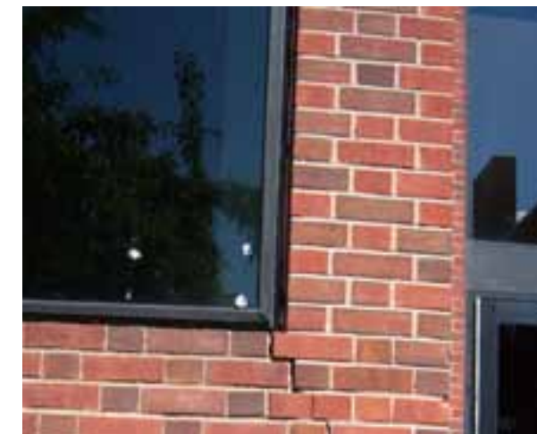
THERE ARE CRACKS IN THE MASONRY ALONG THE BAND OF WINDOWS.
