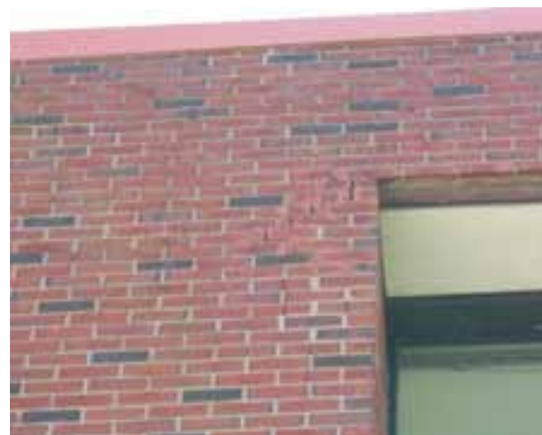
DETERIORATING MASONRY JOINTS.
