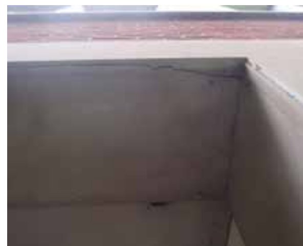
CRACKING IN EXTERIOR CONCRETE LINTEL
