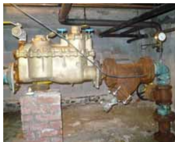
VIEW OF WATER METER
