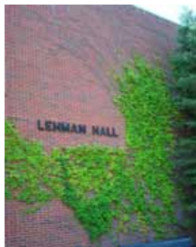
IVY GROWTH ON EXTERIOR MASONRY WALL.
