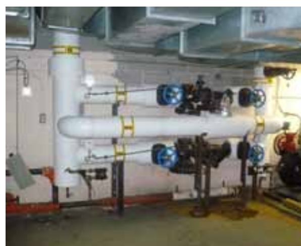
HIGH PRESSURE STEAM ENTRANCE AND PRESSURE REDUCING STATION
