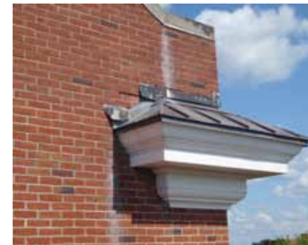
STAINING, SPALLING AND CRACKING OF THE BRICK MASONRY.
