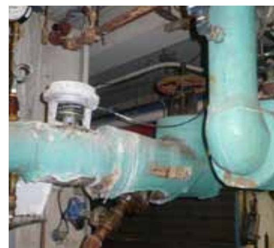
STEAM PIPING AND PRESSURE REDUCING STATION
