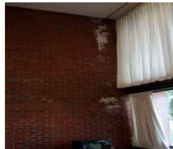
FIRST FLOOR LOUNGE INTERIOR MASONRY STAINING.
