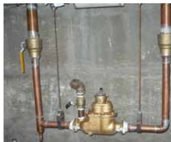
VIEW OF WATER METER
