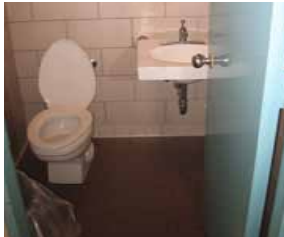
MAINTENANCE FACILITY NON-COMPLIANT TOILET
