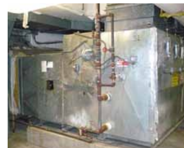
BUILDING AIR HANDLING UNIT
