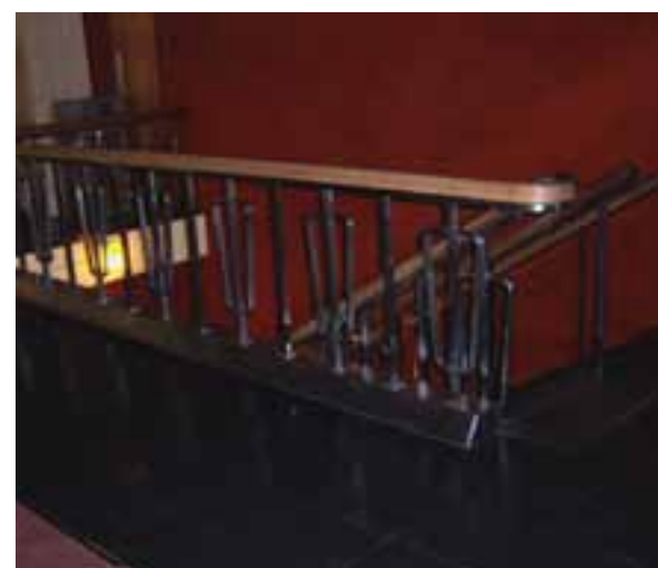
THE COMMUNICATING STAIRWELL
