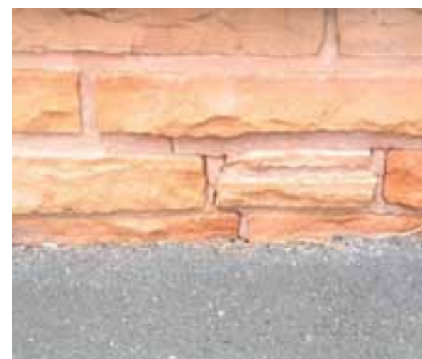
CRACK IN FOUNDATION VENEER MORTAR JOINT.
