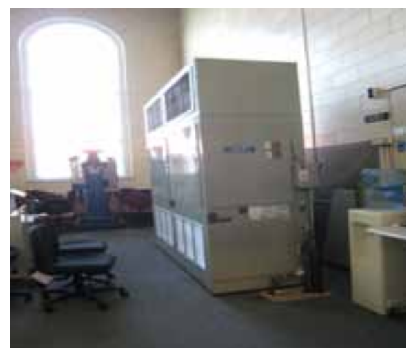
MECHANICAL UNIT LOCATED IN THE CAMPUS' CENTRAL COMPUTER ROOM.
