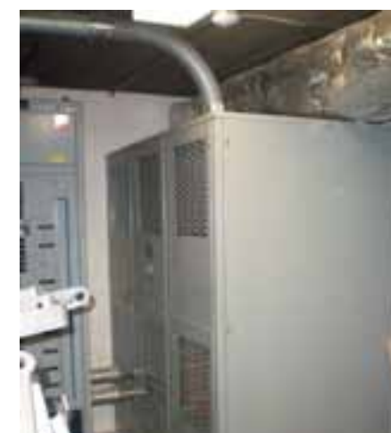
MAIN ELECTRICAL SWITCHGEAR
