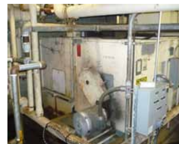
BUILDING AIR HANDLING UNIT
