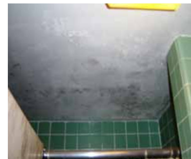
WATER DAMAGE TO CEILING ABOVE SHOWER.
