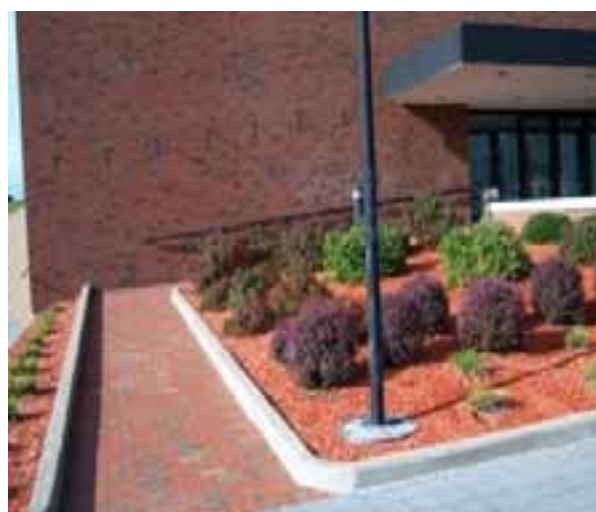
THE RAMP AT THE MAIN ENTRANCE TO THE BUILDING IS MISSING HANDRAILS
