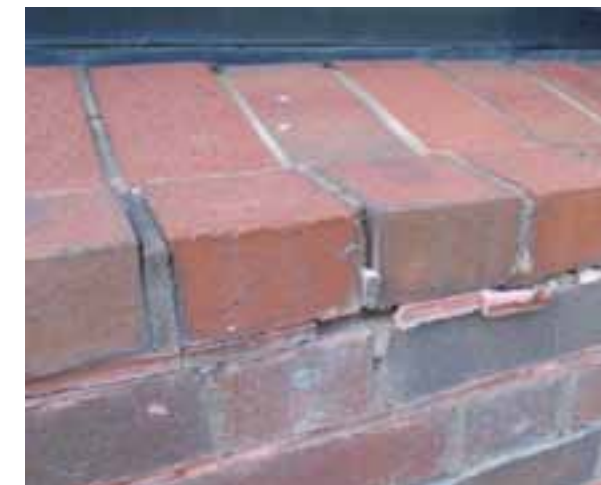
SIGNIFICANT RE-POINTING ISSUES AT THE BRICK SILLS
