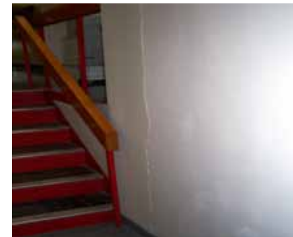
MAJOR CRACK ON THE WALL WHERE THE BUILDING CONNECTS TO CARSON HALL.
