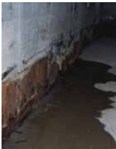
LEAK IN BASEMENT ACCESS ACCESS SPACE BELOW SWIMMING POOL.
