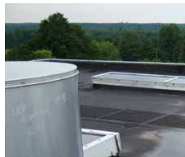
PONDING ON HIGHRISE ROOF
