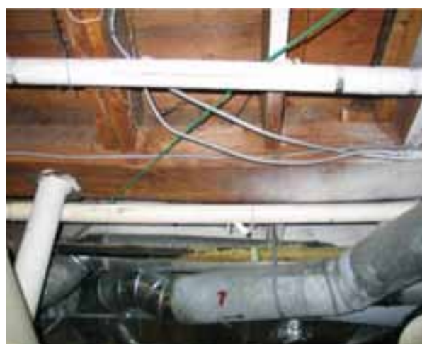
FLOOR BEAM HAS BOWED AT FIRST FLOOR VISIBLE IN THE BASEMENT.
