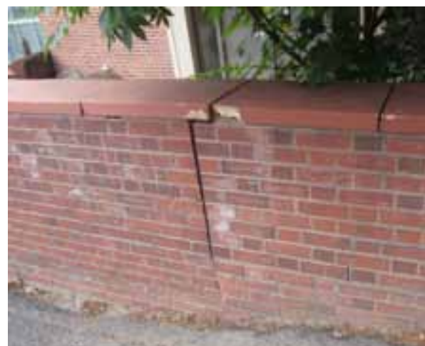
CRACKED RETAINING WALL ON THE EAST END OF THE BUILDING.
