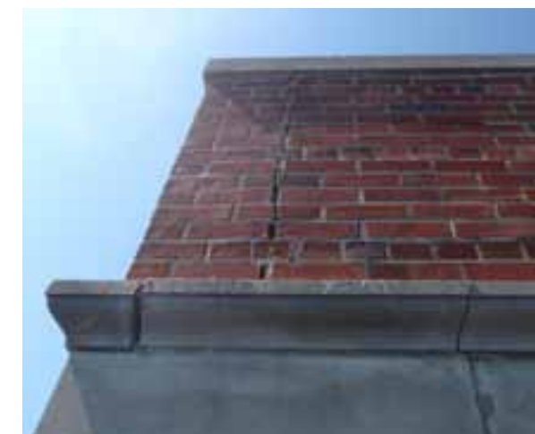
CRACKING OF EXTERIOR MASONRY.
