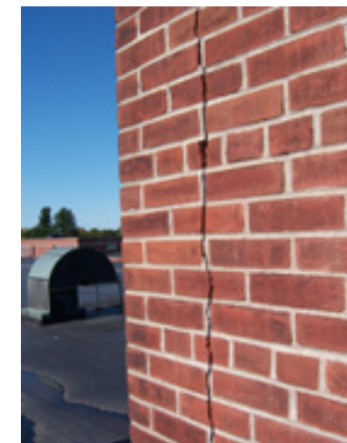
EXTERIOR WALL MASONRY CRACKS.
