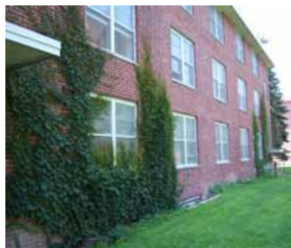
IVY GROWTH ON EXTERIOR MASONRY WALL.
