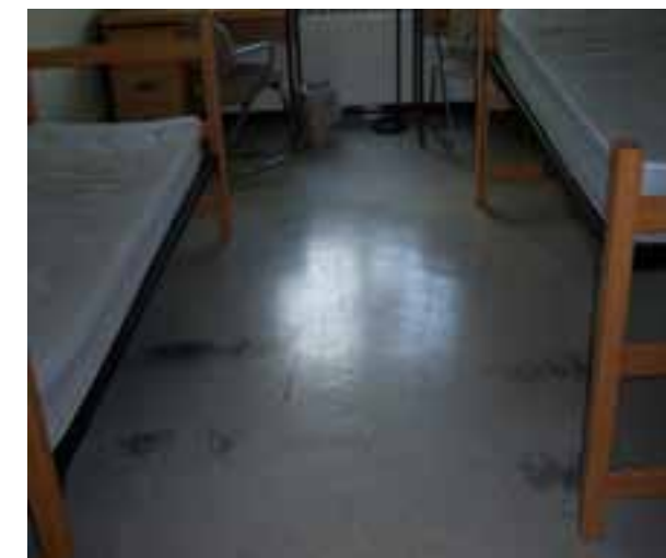
THE FLOOR FINISHES COULD BE REFINISHED TO UPGRADE AESTHETICS.
