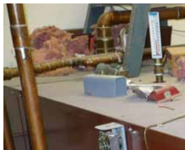
TOP OF AIR HANDLING UNIT
