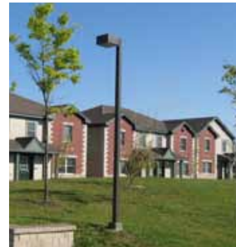
SITE LIGHTING INSTALLATION NEAR TOWNHOUSES
