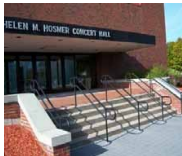
THE MAIN ENTRANCE STAIRS ARE COMPLIANT.
