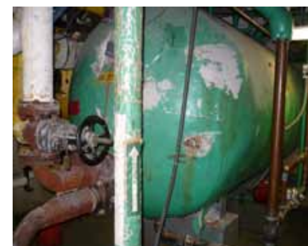
HOT WATER STORAGE TANK
