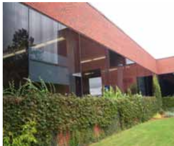
IVY GROWTH ON EXTERIOR MASONRY AND GLAZING WALL.
