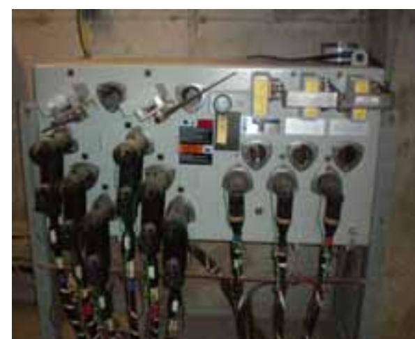
MINA ELECTRIC SERVICE ENTRANCE
