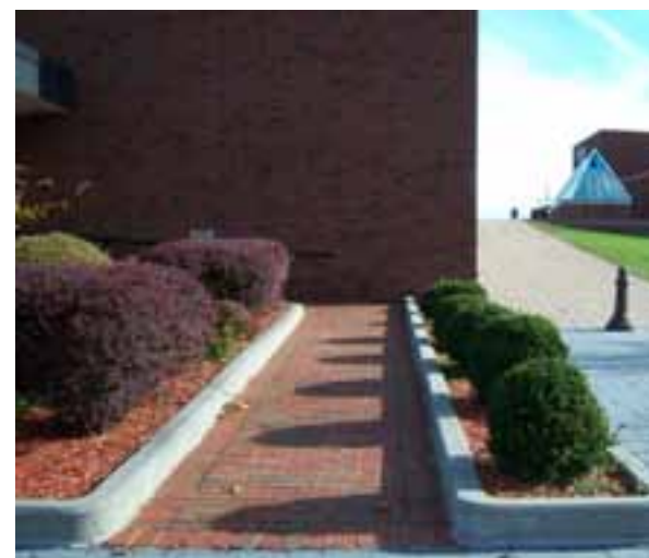
EXTERIOR ENTRY RAMP DOES NOT HAVE HANDRAILS.
