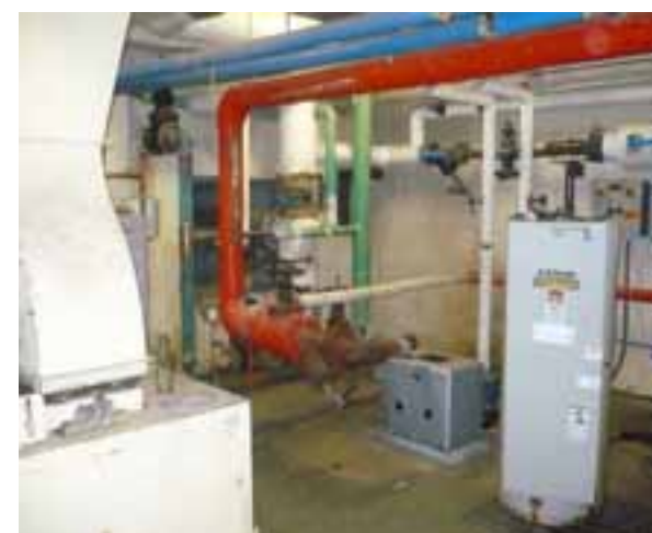
PIPING AND EQUIPMENT IN MECHANICAL ROOM
