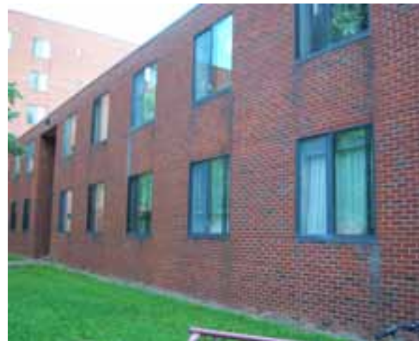
SPALLING AND CRACKS IN THE BRICKS ARE VISIBLE AT SOME LOCATIONS.
