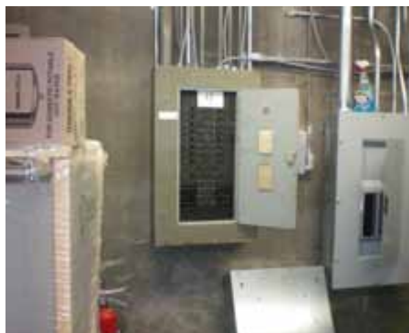
ELECTRICAL PANEL BOARDS
