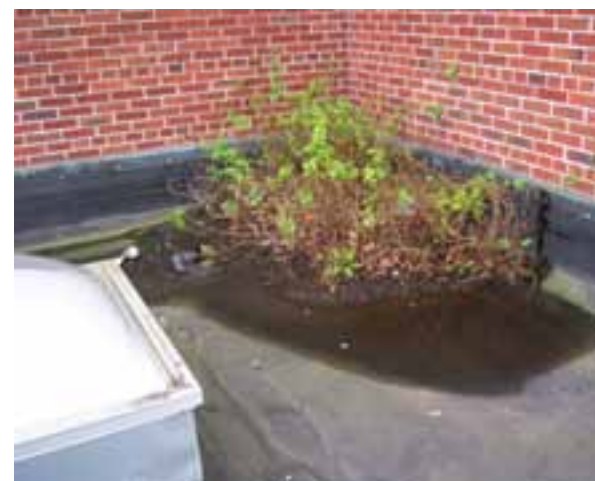
VEGETATION ON ROOF
