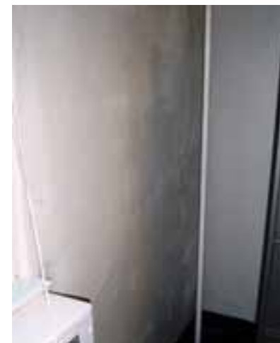
FIRST FLOOR OFFICE
