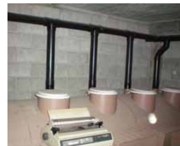
CIVIL DEFENSE TOILET IN AIR-RAID SHELTER
