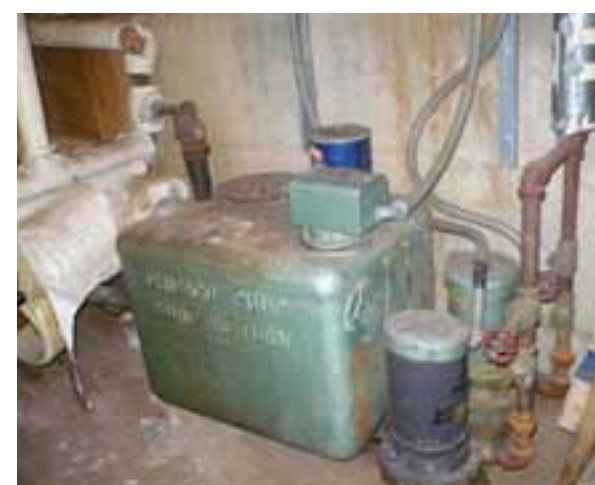
VIEW OF CONDENSATE TANK AND PUMPS
