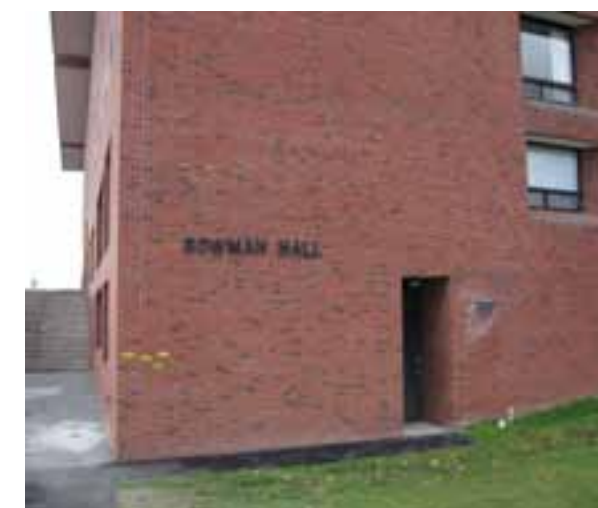
EXTERIOR ENVELOPE MASONRY STAINING.
