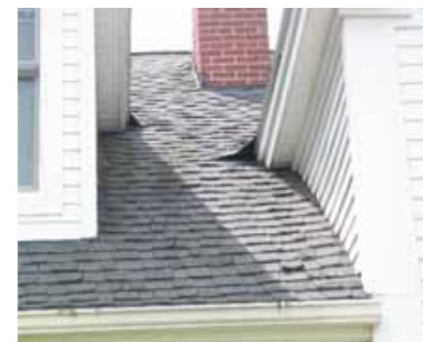
BUILD UP AT PORCH ROOF, AND INSUFFICIENT FLASHING AT CHIMNEY ABOVE.
