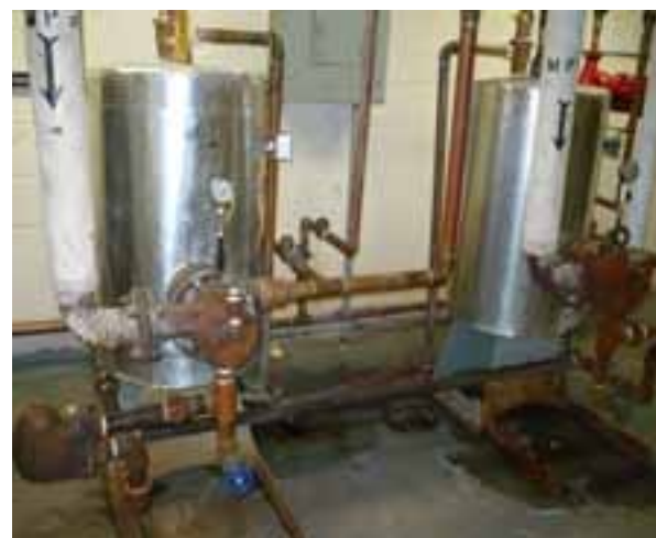
STEAM-TO-HOT WATER CONVERTORS
