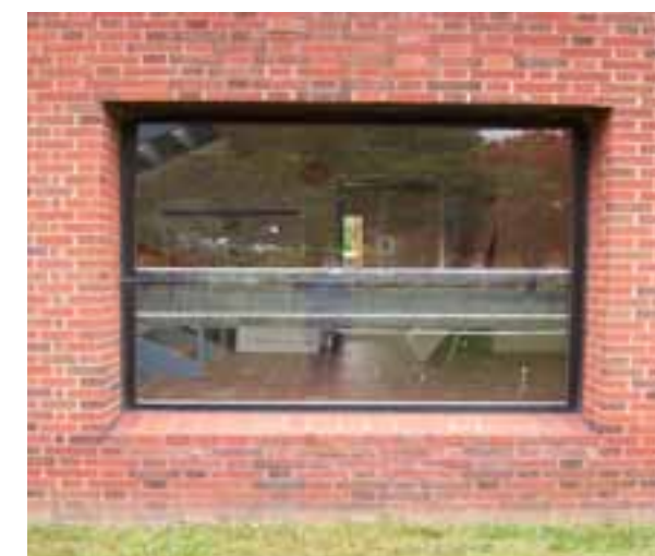
POINTING AND JOINT FAILURE
