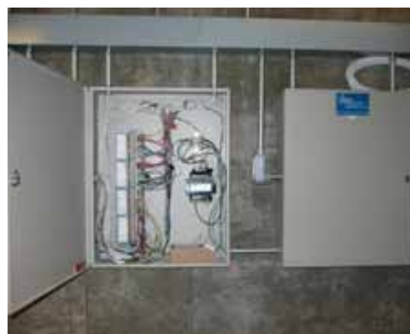
DDC CONTROL PANEL
