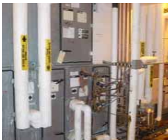
BUILDING AIR HANDLING UNIT
