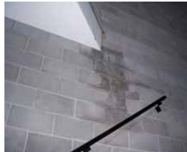
WATER LEAK AT INTERIOR STAIRWELL
