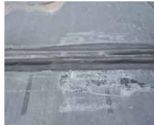
THE FULLY ADHERED EPDM MEMBRANE APPEARS TO BE IN FAIR CONDITION.
