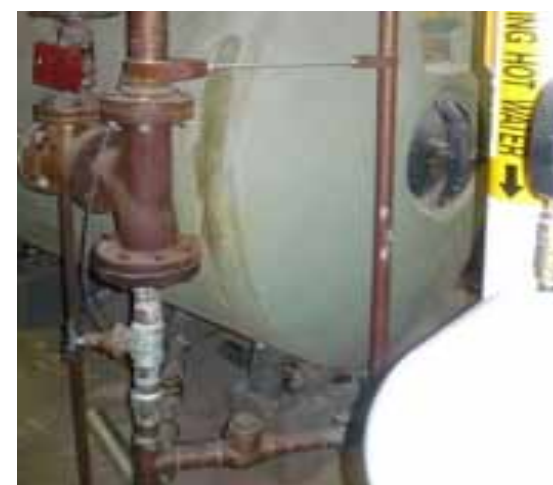
HOT WATER STORAGE TANK
