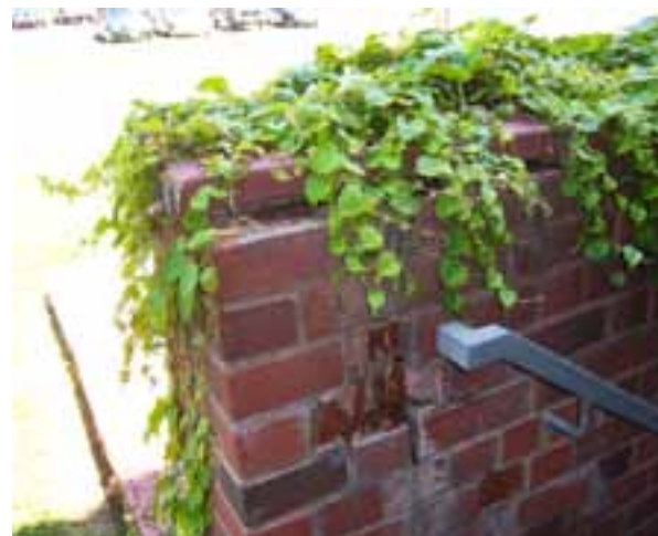
ACCESS STAIR TO THE BASEMENT ON THE WEST SIDE OF THE BUILDING.
