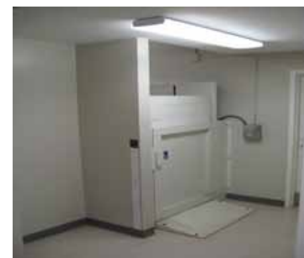
THE WHEELCHAIR LIFT LOCATED AT THE SECOND FLOOR IS NOT ADA-COMPLIANT.
