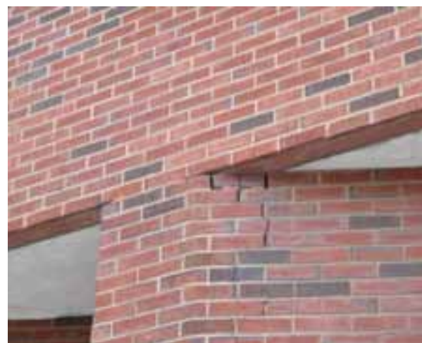
NUMEROUS FRACTURES OF THE MASONRY VENEER.
