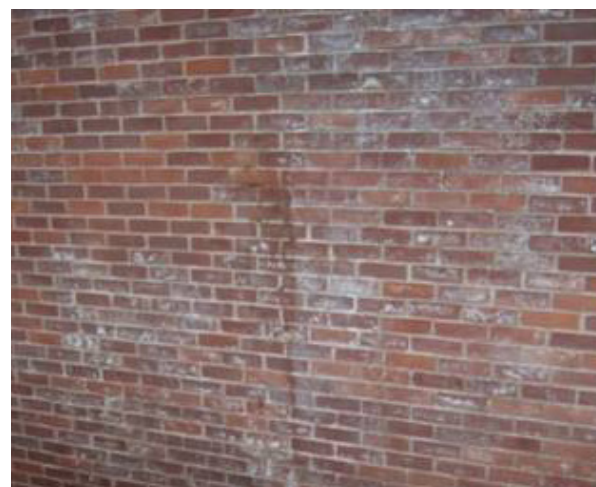
EXTERIOR EFFLORESCENCE EXTENDS TO THE INTERIORS IN SOME AREAS.
