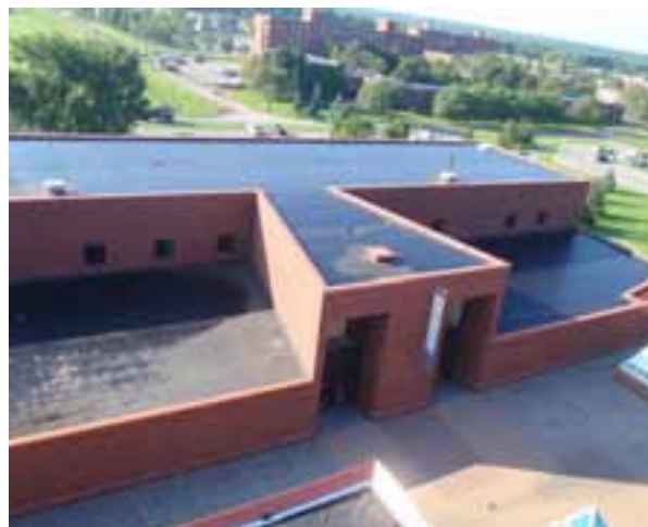
THE ROOF IS IN TWO LEVELS AND IS GENERALLY IN GOOD CONDITION.
