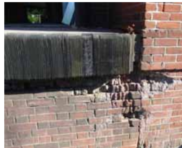
DAMAGE TO BRICK AT LOADING DOCK
