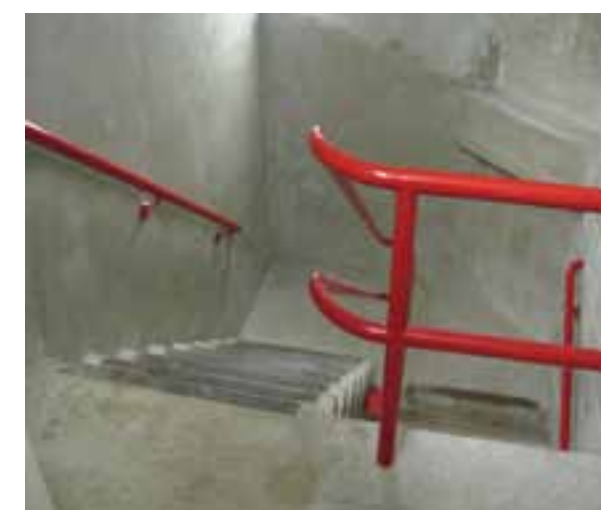
THE STAIRWELLS ARE TOO NARROW AND ARE MISSING GUARDRAILS AND PICKETS.
