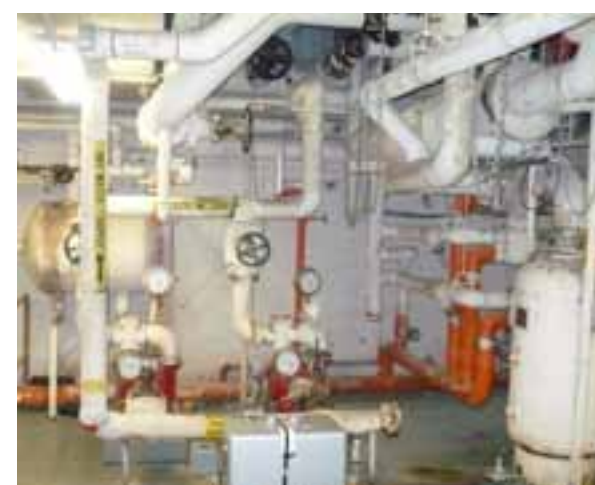
PIPING IN MECHANICAL ROOM
