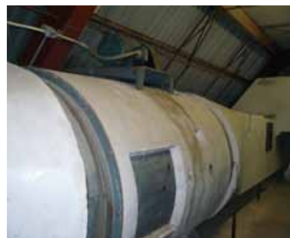
DUCTWORK IN PENTHOUSE
