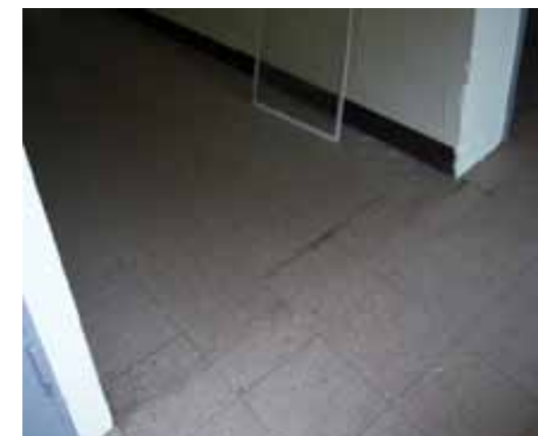
THE INTERIOR FINISHES ARE GENERALLY IN GOOD CONDITION.
