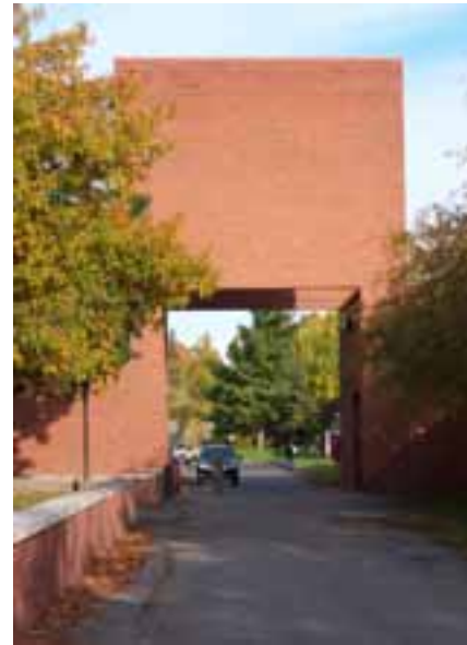
NORTH QUAD TOWER
