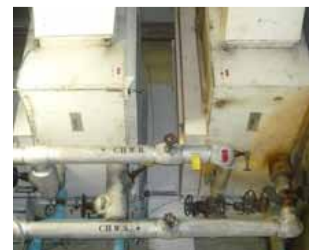
BUILDING AIR HANDLING UNITS
