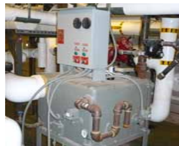
CONDENSATE TANKS AND PUMPS
