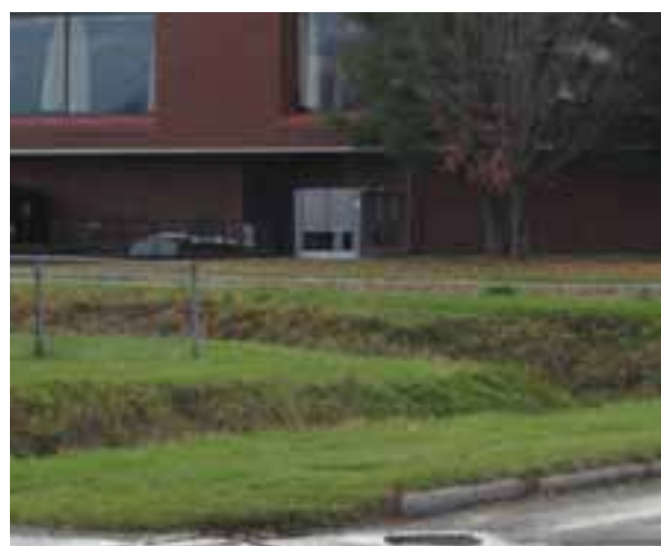
VIEW OF LOADING DOCK
