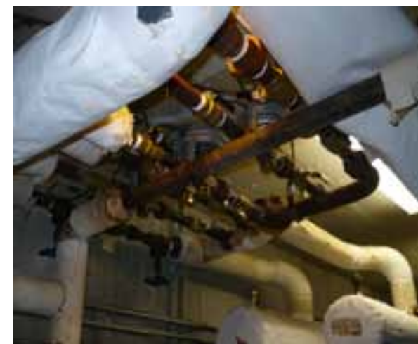
UN-INSULATED STEAM PIPING AND PRESSURE-REDUCING STATION
