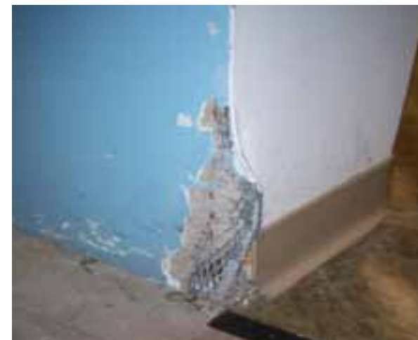
MINOR DAMAGE AND/OR DETERIORATION VISIBLE AT WALLS AT SOME LOCATIONS
