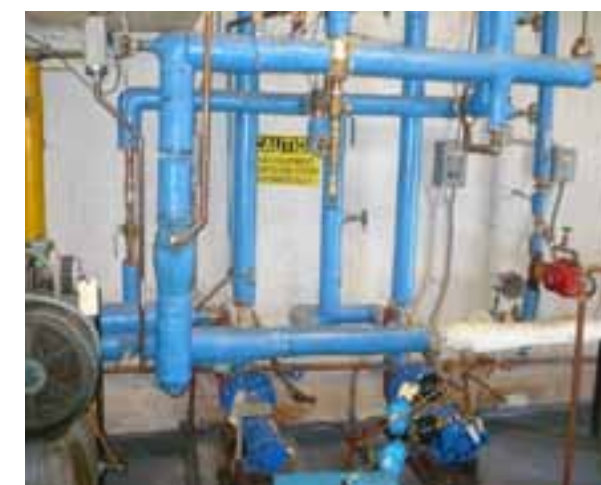
RADIATION ZONE PUMPS
