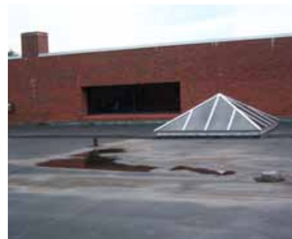
THE SKYLIGHTS HAVE NO FLASHING. TIGHTNESS OF THE GLAZING.
