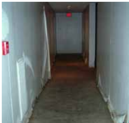
SUBSTANTIAL WATER DAMAGE TO INTERIOR WALLS.
