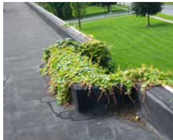
THERE IS SOME VEGETATION GROWTH ON THE ROOFS AND DEBRIS AT THE DRAINS;
