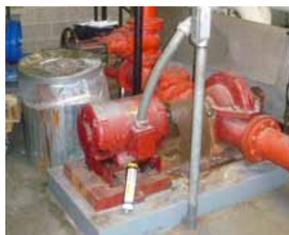
VIEW OF FIRE PUMP
