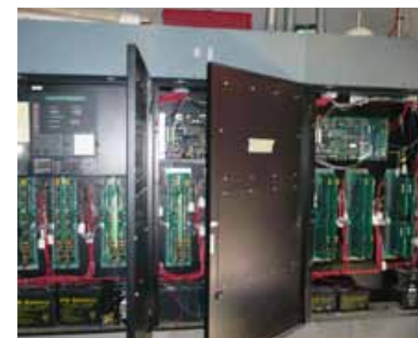
FIRE ALARM PANELS PENTHOUSE
