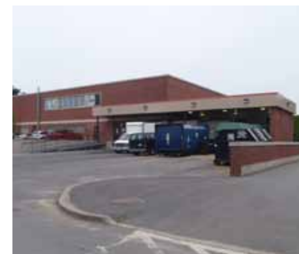
LOADING DOCK AT SOUTHWEST CORNER OF THE BUILDING.
