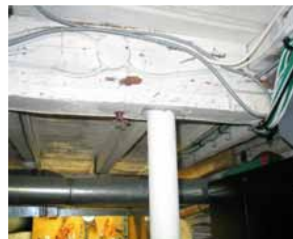
COLUMN LACKS CAP PLATE.
