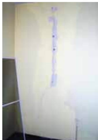
BUILDING CRACKS CAUSED BY MOVEMENT
