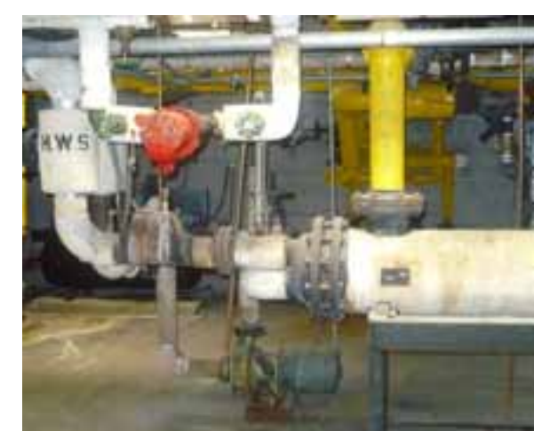
BUILDING HOT WATER CONVECTOR
