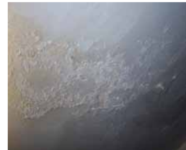
DAMAGE TO THE CEILING IN THE STAIR ROOM.
