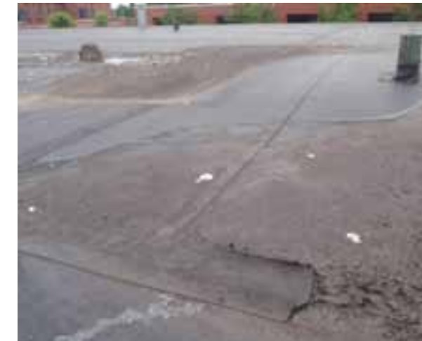
FAILED SEAMS ON THE EPDM ROOF AND DELAMINATED INSULATION
