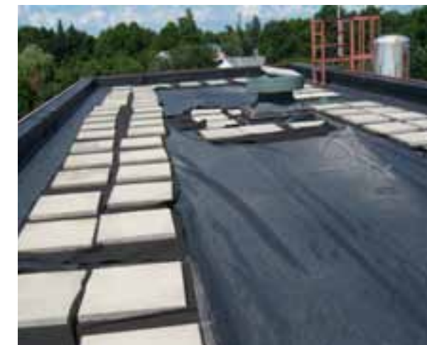
THE EPDM IS NOT ADHERED, RESULTING IN THE MEMBRANE FLAPPING IN THE WIND.
