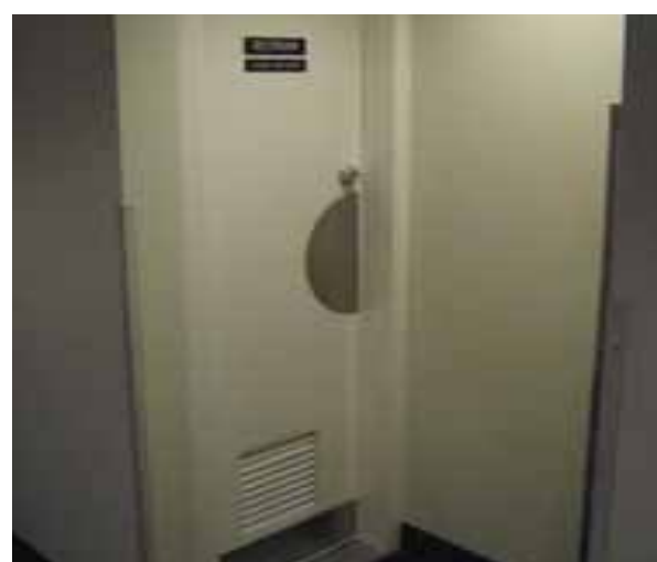
PUBLIC RESTROOM DOORS ARE TOO NARROW FOR WHEELCHAIRS.
