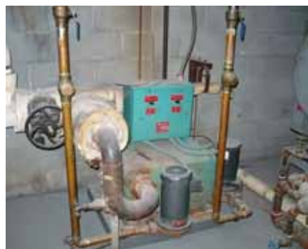
CONDENSATE TANK AND PUMPS
