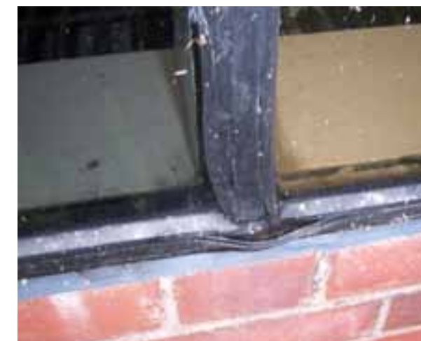
WINDOW FRAME IN POOR CONDITION
