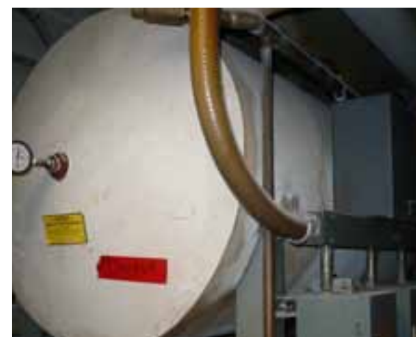
HOT WATER TANK
