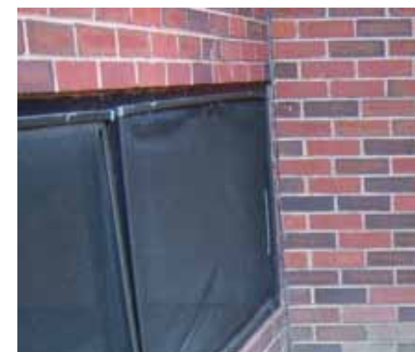
POOR MASONRY BASE
