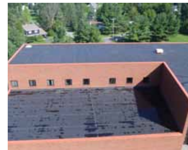
ROOF IS GENERALLY IN GOOD CONDITION.
