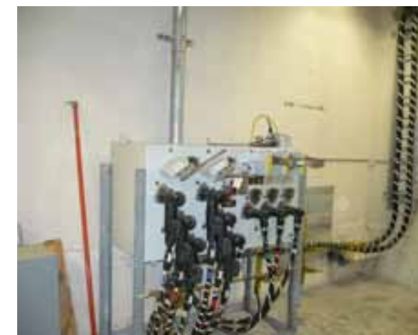
MAIN ELECTRICAL SERVICE ENTRANCE
