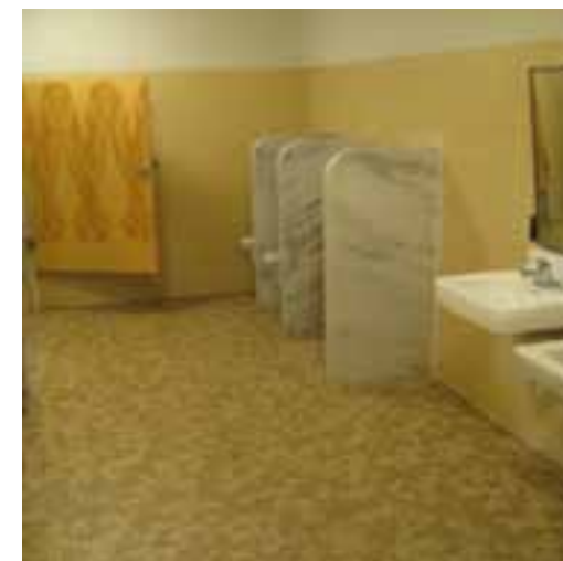
THE FIRST FLOOR TOILET ROOMS ARE 90% COMPLIANT
