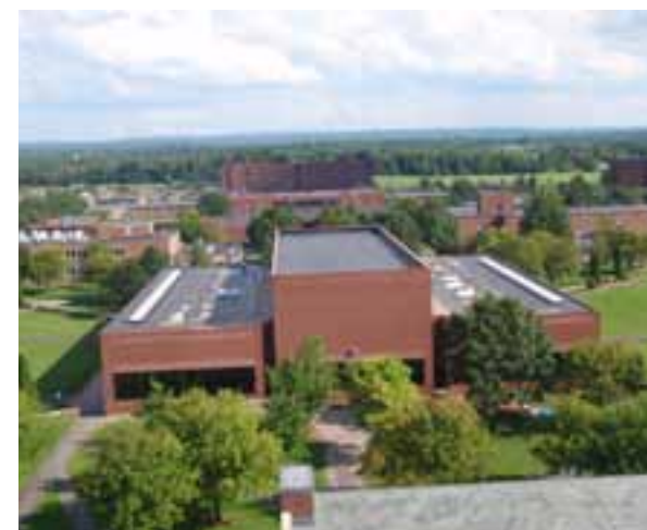
THE LOWER ROOFS REQUIRE ATTENTION IN SOME AREAS.
