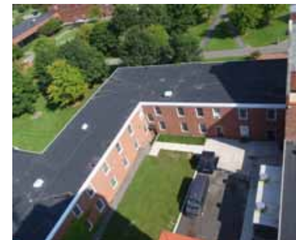
EPDM MEMBRANE IS GENERALLY IN GOOD CONDITION.
