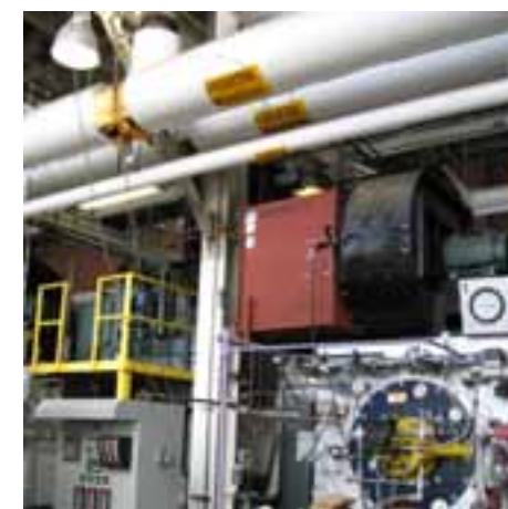
VIEW OF BOILER BURNER
