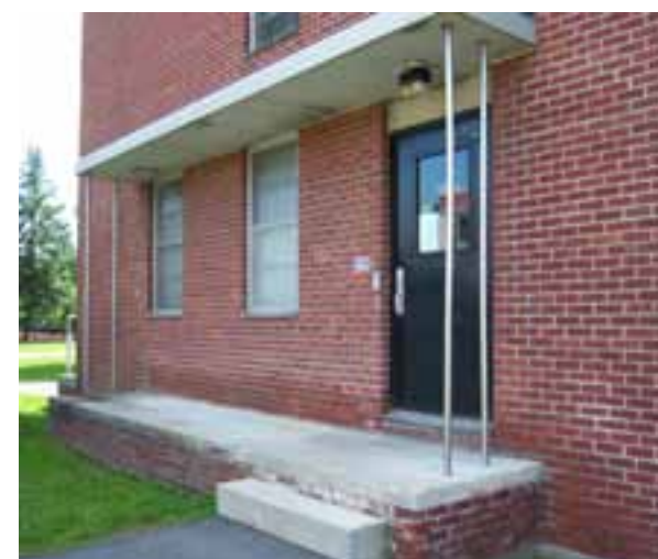
ENTRANCE IS NOT WHEELCHAIR ACCESSIBLE.
