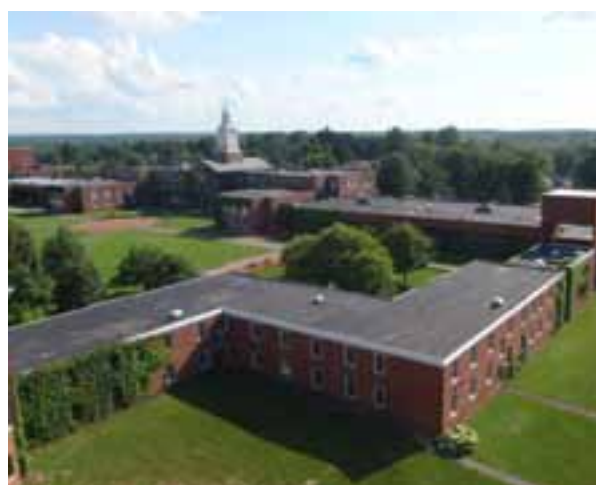
VIEW OF ROOFTOP.
