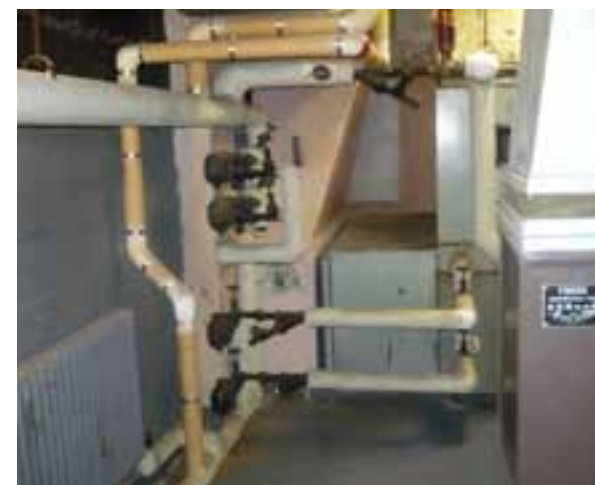
BUILDING AIR HANDLING UNIT
