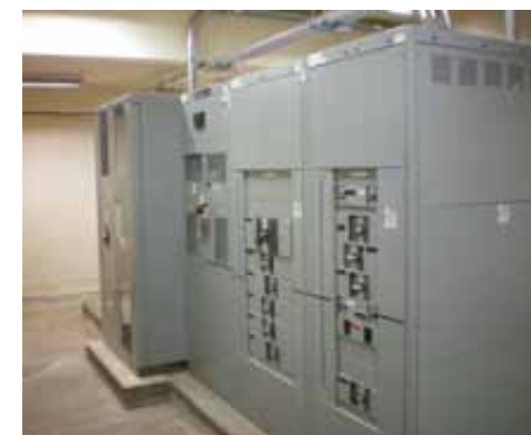
MAIN ELECTRICAL SWITCHGEAR
