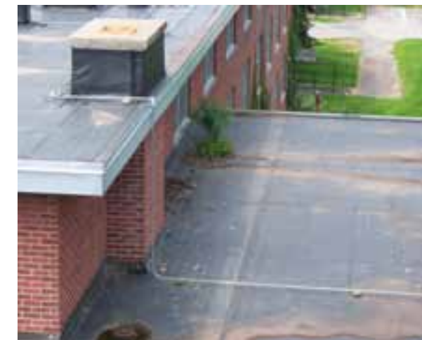
VEGETATION ON LOW ROOF.
