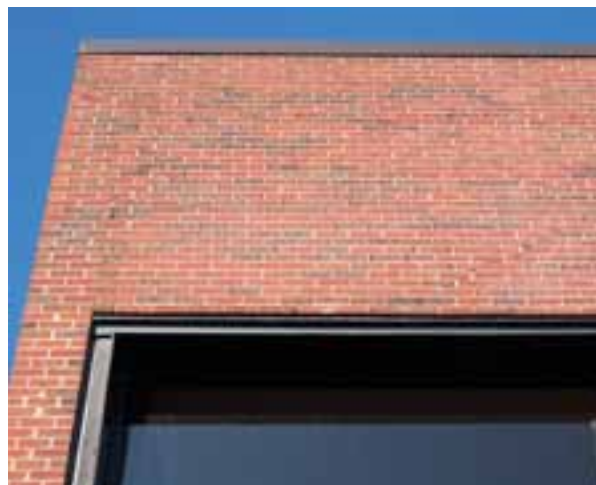
CRACKS IN EXTERIOR MASONRY.
