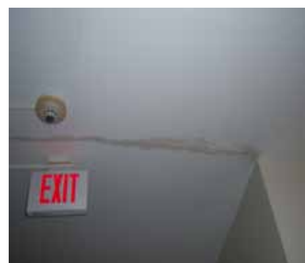
CRACK IN CORRIDOR CEILING AT CARSON HALL AND MACVICAR CONNECTION
