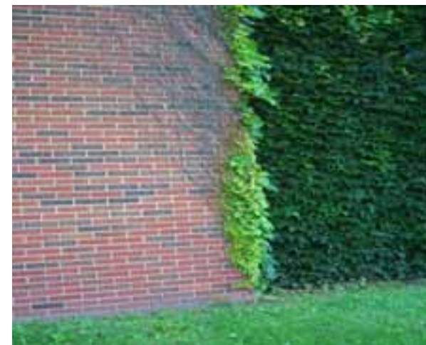
IVY GROWTH ON EXTERIOR MASONRY WALL.
