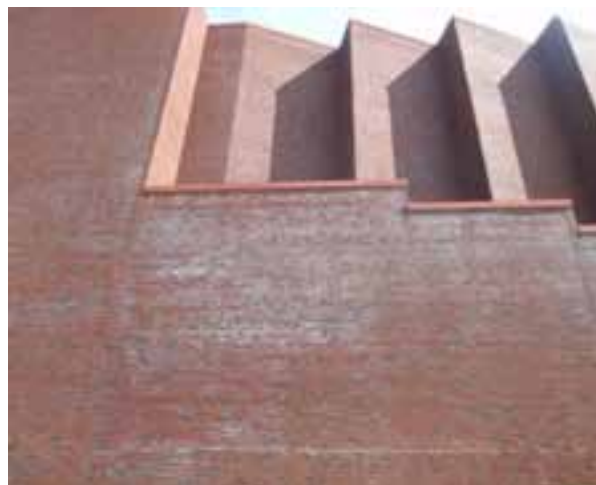
EXTERIOR ENVELOPE EFFLORESCENCE & STAINING
