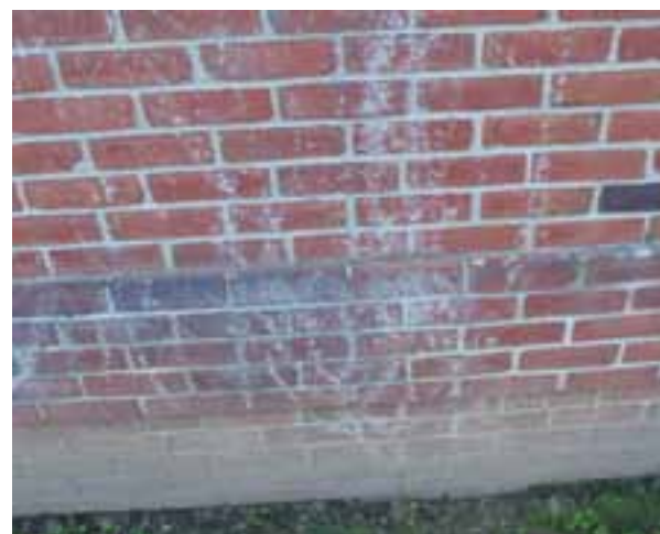
EFFLORESCENCE OCCURRING AT EXTERIOR MASONRY.
