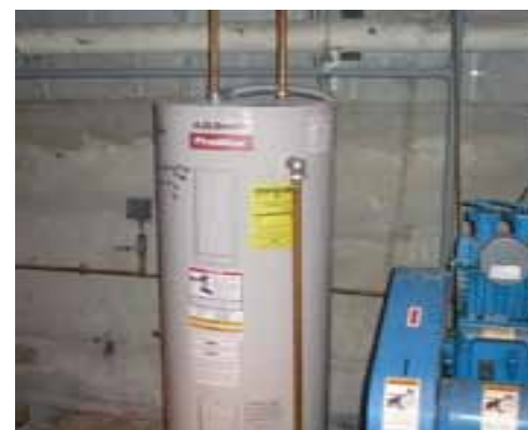
ELECTRIC WATER HEATER
