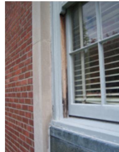
WINDOW AND GLAZING MAINTANENCE.
