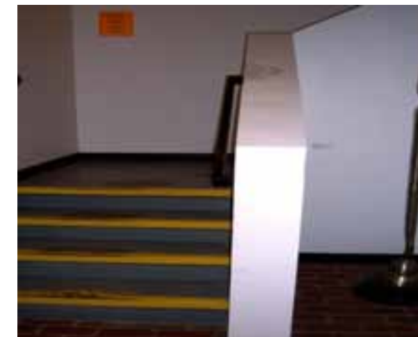
VIEW OF BUILDING WORN FINISHES
