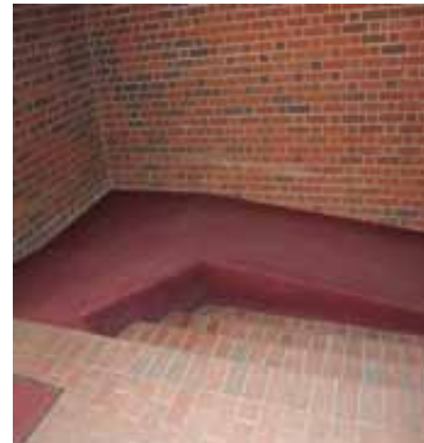
NON-COMPLIANT RAMP IN MER- RITT HALL
