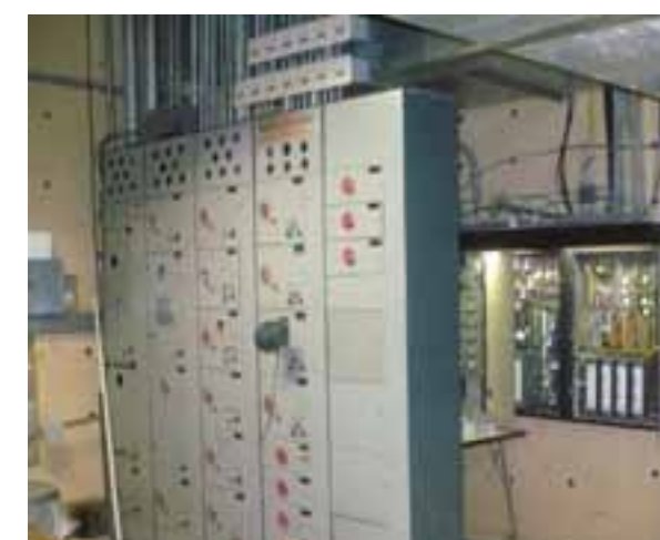
CRANE COMPLEX: MOTOR CONTROL CENTER
