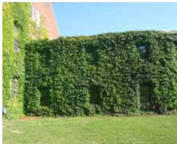
SEVERE IVY GROWTH ON EXTERIOR BUILDING ENVELOPE.
