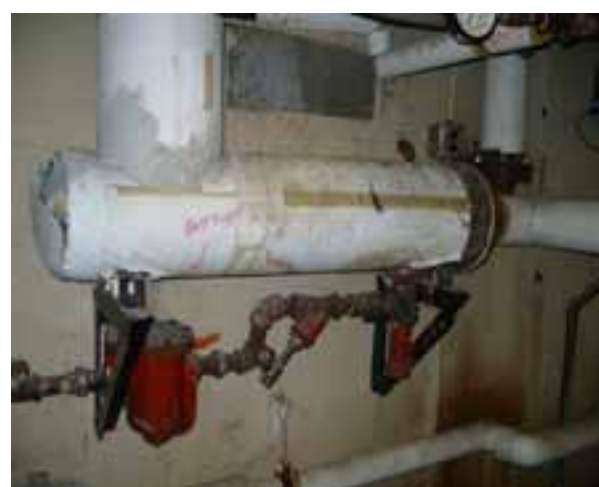
HOT WATER CONVERTOR
