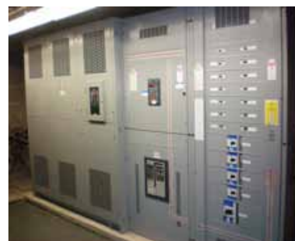
MAIN ELECTRICAL SWITCHGEAR
