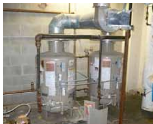
NATURAL GAS-FIRED HOT WATER HEATERS
