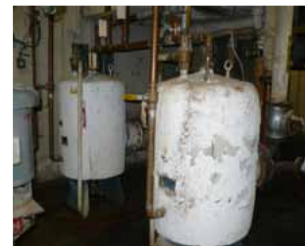
STEAM-TO-HOT WATER CONVERTORS
