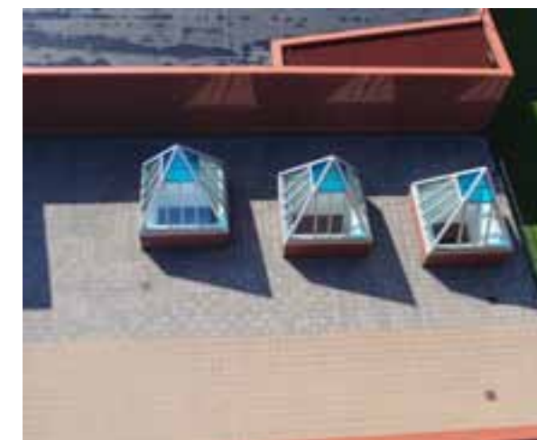
THE ROOF IS THE PLAZA. IT IS PAVED WITH SQUARE ASPHALT PAVERS.
