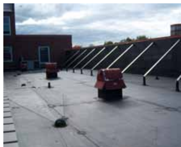
ROOF DRAINS AND EXHAUST FANS
