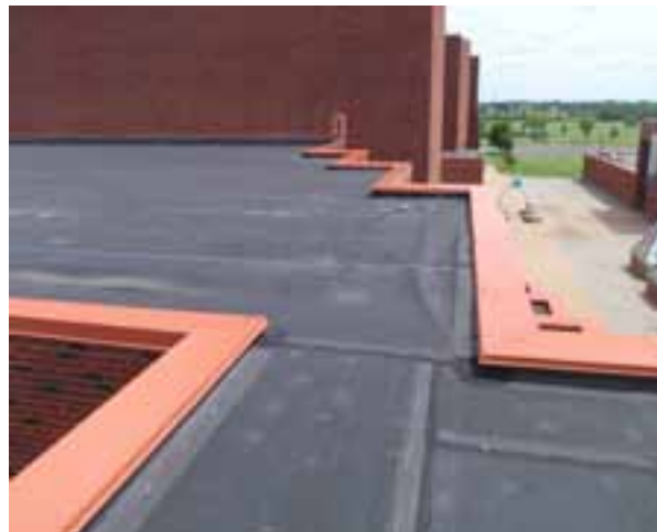
THE EPDM IS POOR ON ONE OF THE NORTH LOWER ROOFS OF THE BUILDING.
