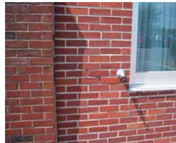
MASONRY JOINTS REQUIRE RE-POINTING AT MANY LOCATIONS.
