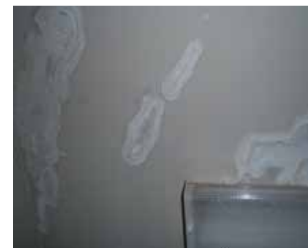
MOISTURE DAMAGE ON PLASTER WALLS.
