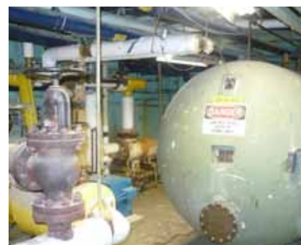
HOT WATER STORAGE TANK AND STEAM PIPING
