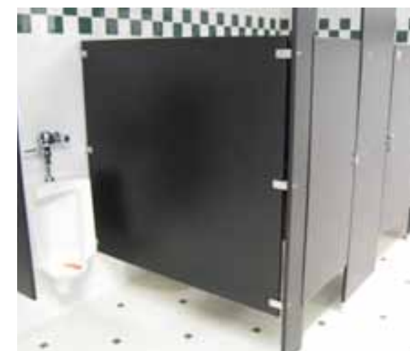
RECENTLY RENOVATED TOILET ROOM.
