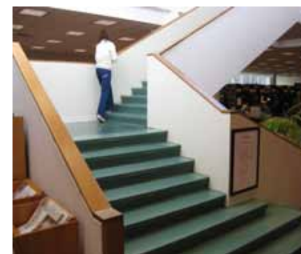
THE MAIN COMMUNICATING STAIR DOES NOT HAVE HANDRAILS.
