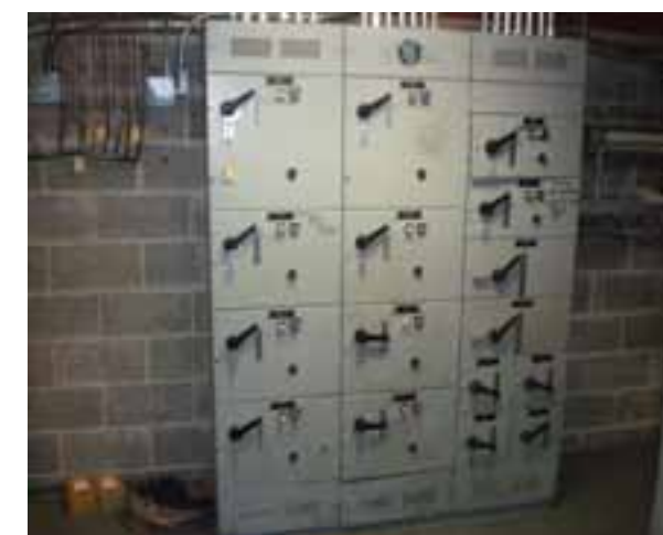
MOTOR CONTROL CENTER
