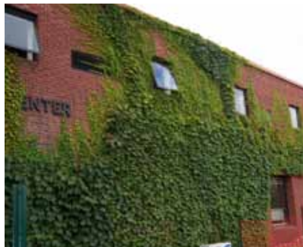
IVY GROWTH ON EXTERIOR ENVELOPE
