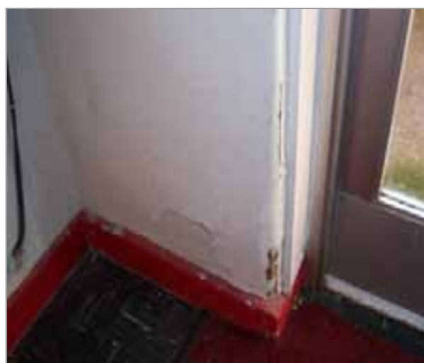
DAMAGE AT INTERIOR WALLS
