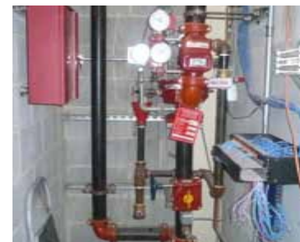
PRE-ACTION SPRINKLER VALVE AND PIPING
