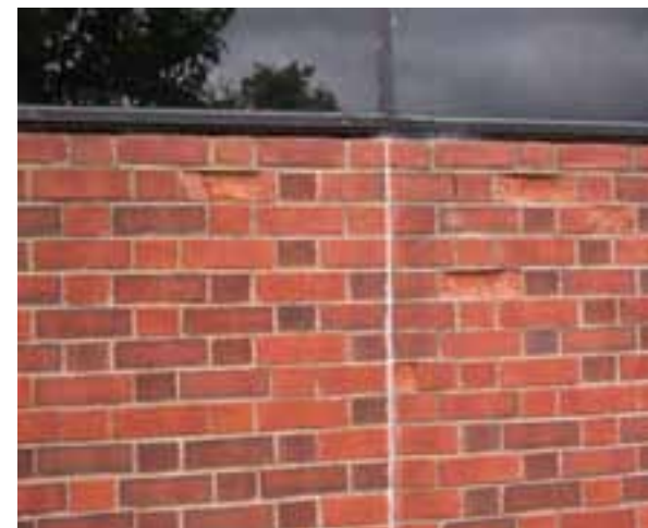
BRICK SPALLING AND DETERIORATED GROUT JOINTS ON THE EAST SIDE.
