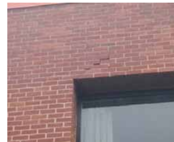
LARGE DIAGONAL CRACKS IN THE MASONRY AT THE LINTELS DUE TO MASONRY MOVEMENT AND EXPANSION.
