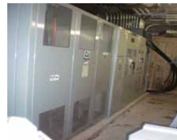
MAIN ELECTRICAL SWITCHGEAR
