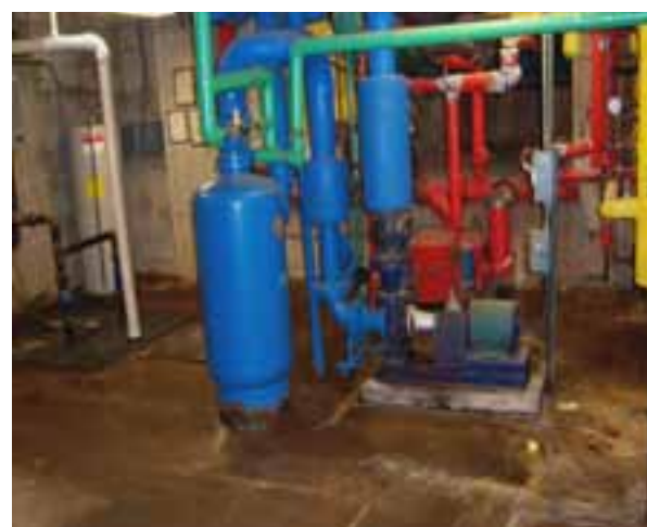
HEATING HOT WATER PIPING AND PUMPS
