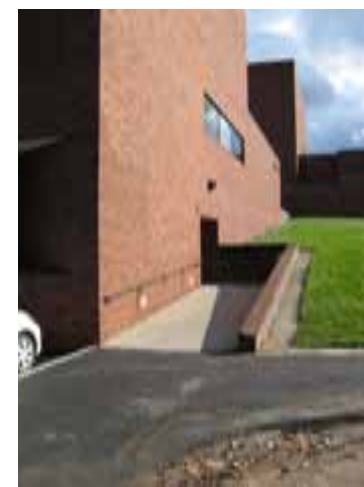
EXTERIOR RAMP DOES NOT HAVE HAND-RAIL EXTENSIONS.
