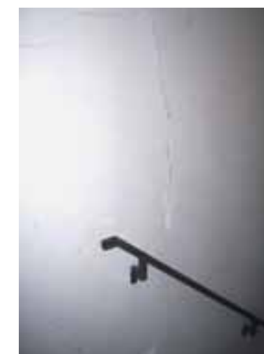
THE EGRESS STAIRWELLS ARE MISSING HANDRAIL EXTENSIONS.
