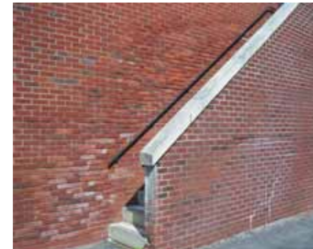
THE MASONRY WALL ENCLOSURE AT THE EXTERIOR STAIR IS IN POOR CONDITION
