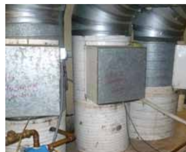
CRANE COMPLEX: UNDERGROUND DUCTWORK FROM AIR HANDLING UNITS
