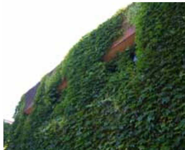
IVY GROWTH ON EXTERIOR MASONRY WALL.
