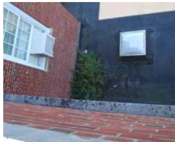
VEGETATION ON LOWER ROOF
