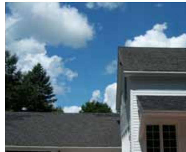
THE ROOF SHINGLES ARE FAIR TO POOR CONDITION.
