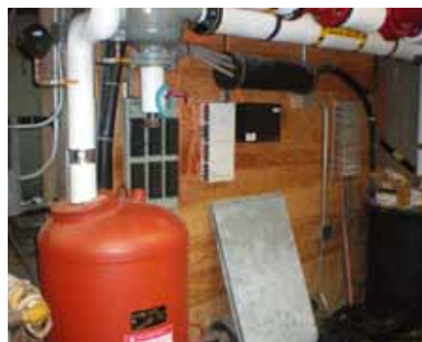
VIEW OF EXPANSION TANK
