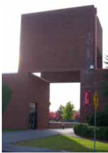
WEST QUAD TOWER
