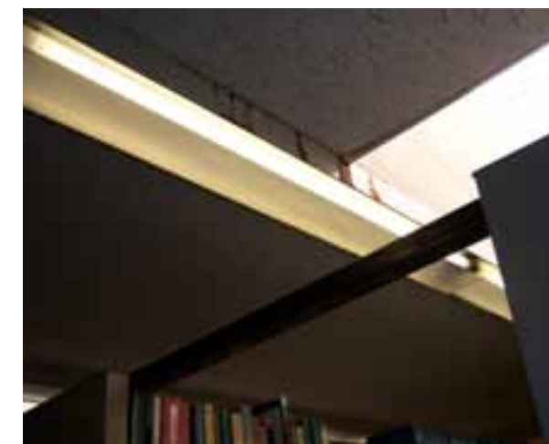
WATER LEAK AT SKYLIGHT.
