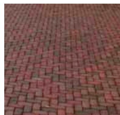
PERMEABLE COMPOSITE PAVERS
