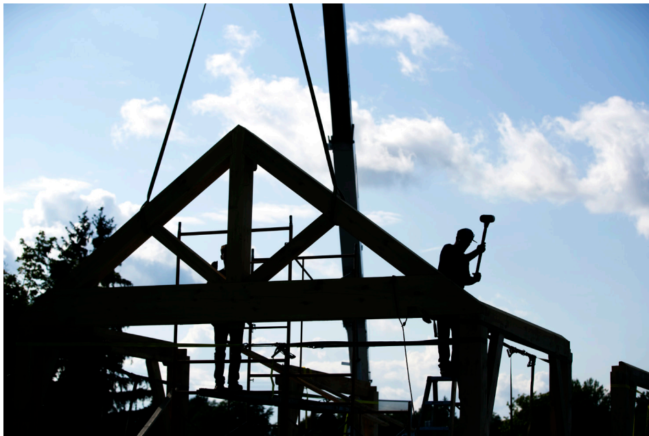
Construction of HEARTH (Photograph by Jason Hunter).
